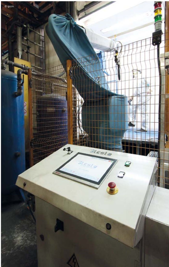
Ideal System is currently testing the implementation of a pair of Lesta articulated robots on its powder coating booth.
