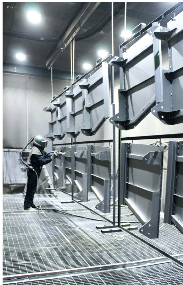
Vespa Sabbiatrici's manual blow-off and sandblasting chamber placed in line with the shot blasting machine.
